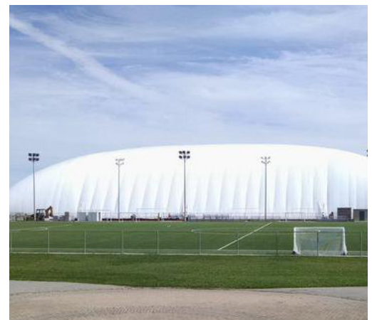
Left: Canopy and seating; Right: Domed soccer field
