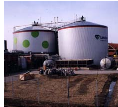
Figure 6.12: Biogas can be generated from decomposing agricultural wastes and used for the generation of heat and electricity. Biogas is a natural, renewable resource that has the added benefit of diverting wastes from the landfill – Biogas Collection Facility, Sweden
