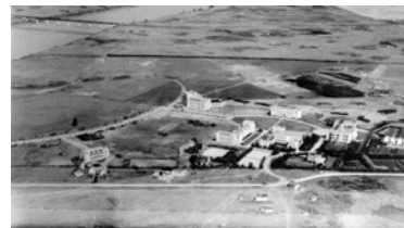
Figure 2.4: 1928 aerial view showing the partial realization of the original 1909 Master Plan
