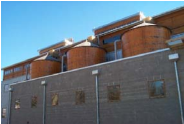
Figure 6.11: Cisterns can collect and store rainwater from rooftops for later use in irrigating landscapes and crops – Chesapeake Bay Foundation, Annapolis Maryland
