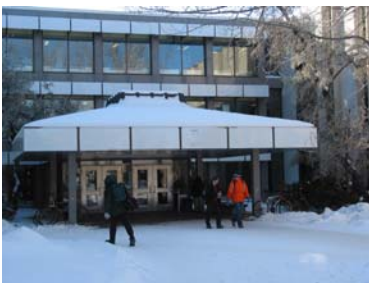
Figure 4.14: Canopies serve as a protective element at ground level – University of Saskatchewan
