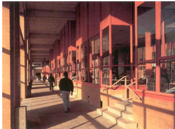
Figure 4.15: Colonnades serve as a protective element at ground level, sheltering people from wind, rain and snow – York University
