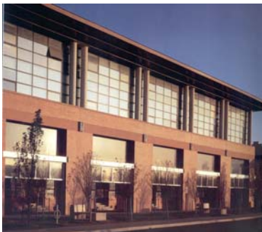
Figure 4.6: Active building and pedestrian pathways are visually and physically connected – York University
