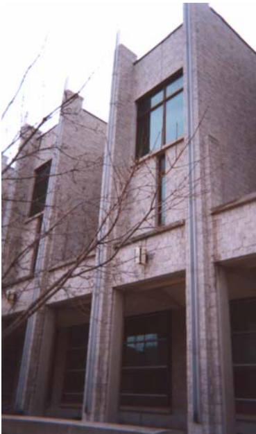
Figure 4.13: Higher floors are expressed with building envelope variation – Queen's University
