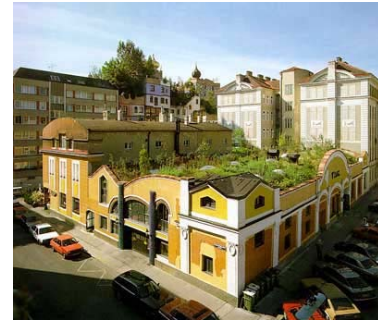
Figure 6.9: Vegetated roofing systems can help to reduce and filter peak storm-water loads, remove airborne particles and carbon dioxide from the air, guard against urban heat island effect and reduce the costs associated with heating and cooling the building – Kalke Village Shopping Centre, Vienna, Austria
