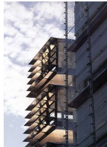
Figure 6.6: Sun louvers can help to reduce large solar gains, cooling the interior of the building – Computer Technology Building, Austria
