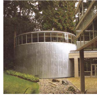
Figure 4.25: Lui Centre at University of British Columbia was required to meet a high standard of energy efficiency
