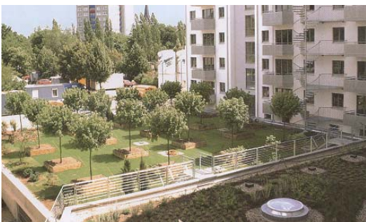
Figure 4.27: Using drought resistant landscaping strategies including the use of grey water and rainwater can reduce the need for irrigation systems
