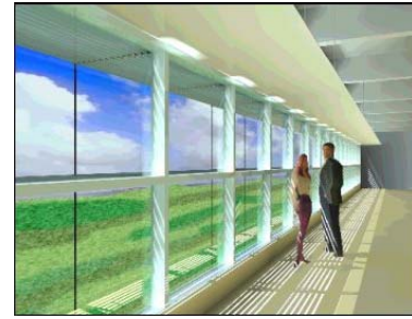
Figure 6.5: Light shelves can be used to bounce light further into the interior of the building. Using daylight to provide illumination is both environmentally friendly and cheap – BC Gas Operations Centre, Surrey, BC
