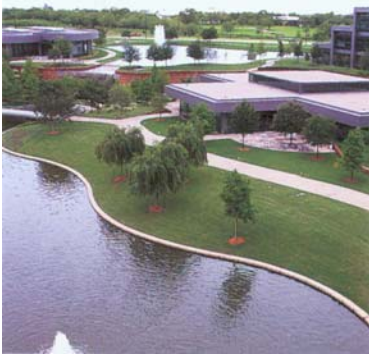
Figure 6.10: Stormwater management can help to increase soil infiltration of storm-water, treat and reduce peak flows and add visual interest and variety to the landscape
