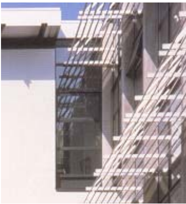
Figure 4.30: Shading louvers on southern exposures reduces heat gain in the summer
