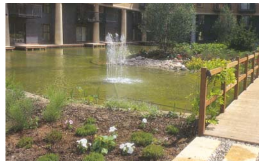
Figure 4.28: Storage of rainwater in retention ponds controls runoff
