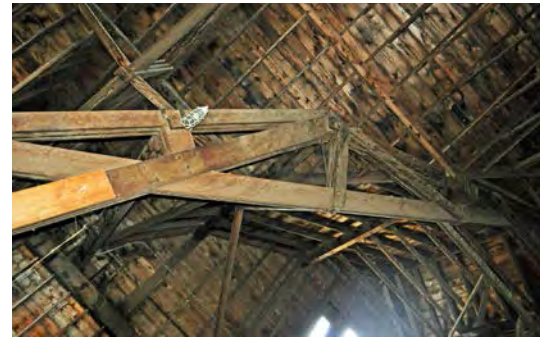
Figure 18. The structure of the barn roof.
