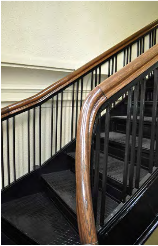
Figure 6. The uppermost staircase: iron treads, stringers and balustrade, oak banister.
