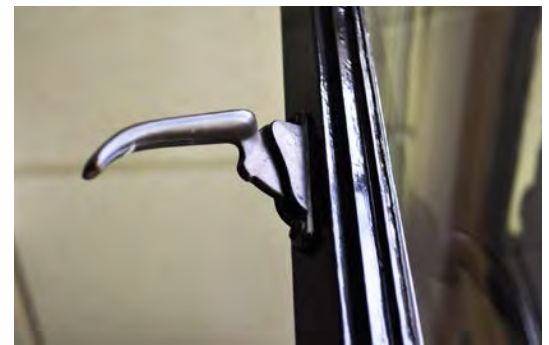
Figure 5. L to R: brass window clasp, painted steel sash window.
