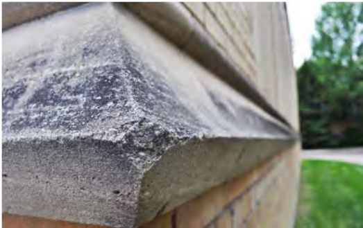
Figure 2. Limestone string course.
