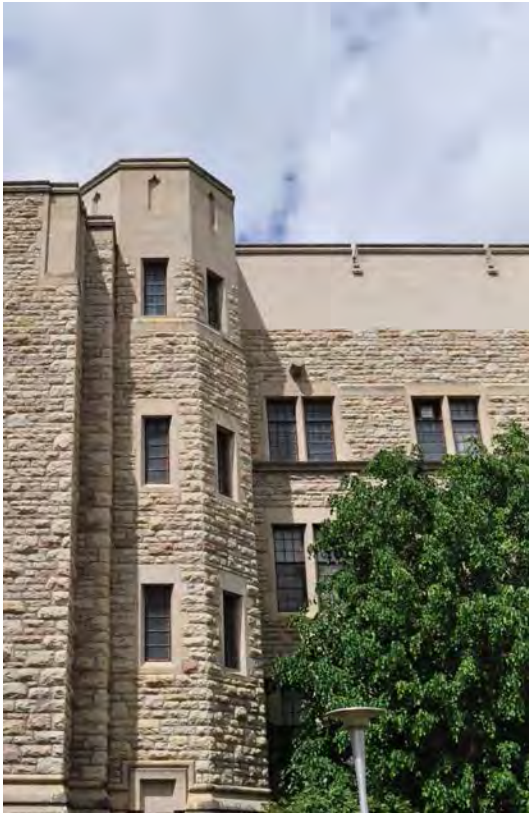
Figure 14. Octagonal stair tower.
