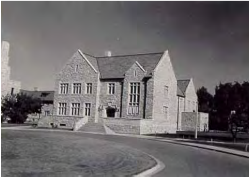
Figure 3. The Memorial Union Building, 1958. Photo A-563, retrieved from http://sain.scaa.sk.ca/items/index.php/memorial-union-building-exterior-13;rad .
