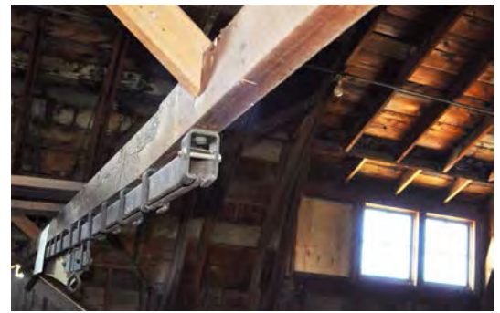
Figure 16. Steel rail & pulley system attached to wood beam.
