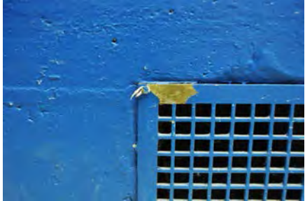
Figure 10. Concrete wall and brass grille that have been painted.
