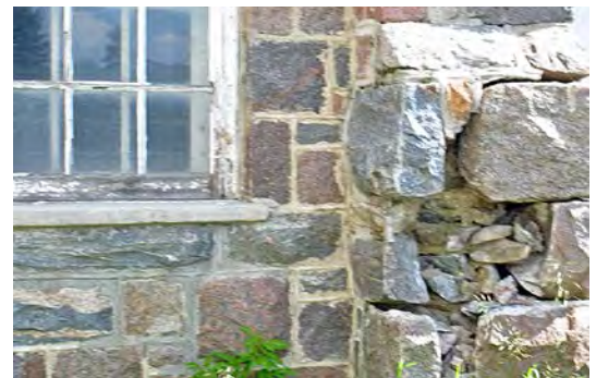
Figure 4. Ground floor walls are constructed of red and grey, rough-faced granite. Windows are framed in wood.
