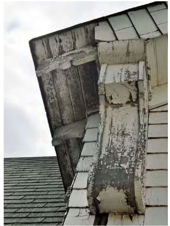
Figure 12. Carved wooden brackets flank the ramp doorway and carved wooden rafter extensions are visible under the eaves.
