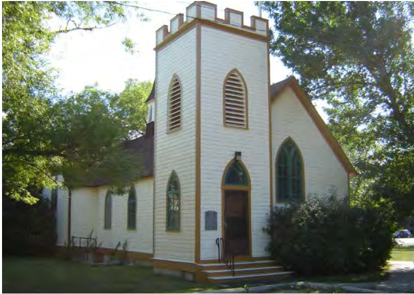
Figure 2. Rugby Chapel from the north-east.
