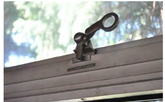
Figure 13. Aluminum window frame and steel handle.
