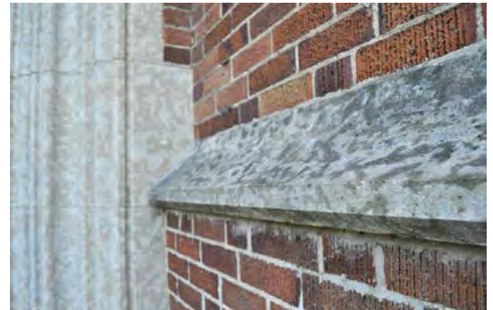
Figure 13. Tyndall stone string course.
