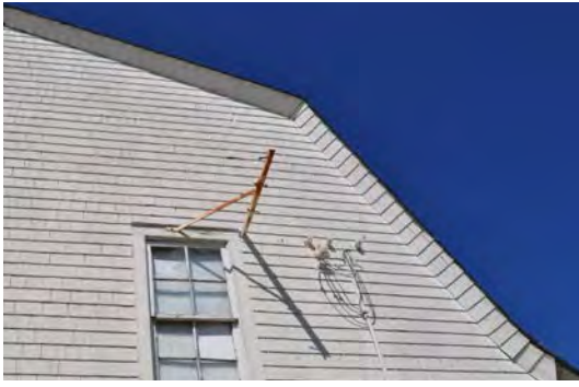
Figure 7. The distinctive slope of the Gambrel style roof.
