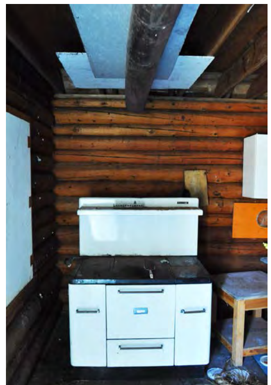
Figure 17. Original wood-burning stove.
