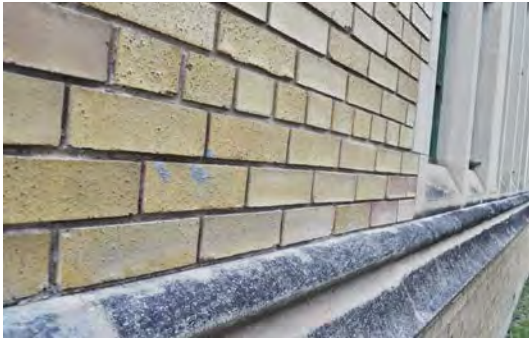
Figure 16. Limestone string courses and window surrounds.
