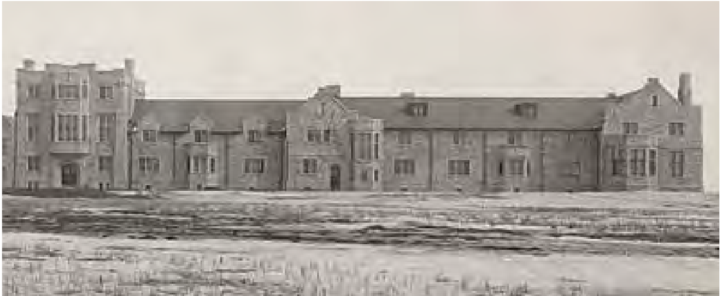
Figure 16. An elevational view of Saskatchewan Hall from the west. Photo A-27, retrieved from http://sain.scaa.sk.ca/items/index.php/?search?page=2&query=a-27&limit=10 .
