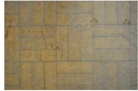
Figure 10. Patterned concrete tile.
