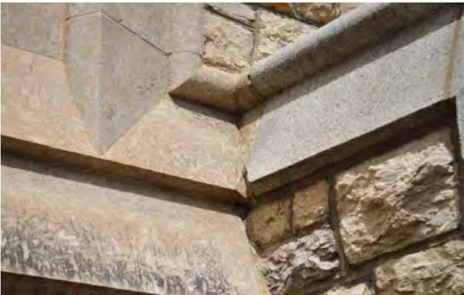
Figure 1. Stone materials: greystone and Tyndall stone.
