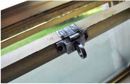
Figure 7. Gold anodized aluminum window frame, with steel hardware.
