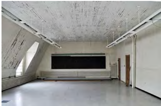
Figure 16. The first floor lecture hall.
