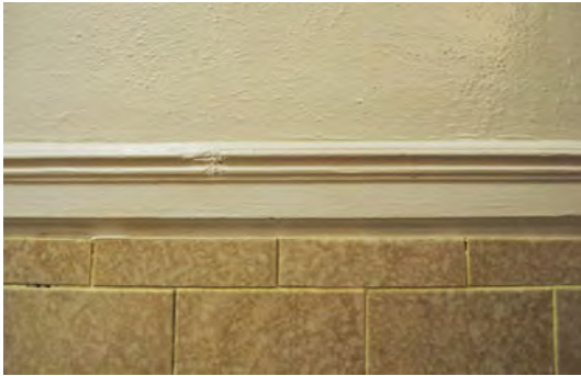
Figure 8. Plaster wall with painted wooden dado and glazed tile wainscoting.
