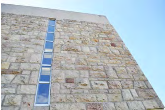
Figure 25. Narrow windows make reference to historical archer slots.
