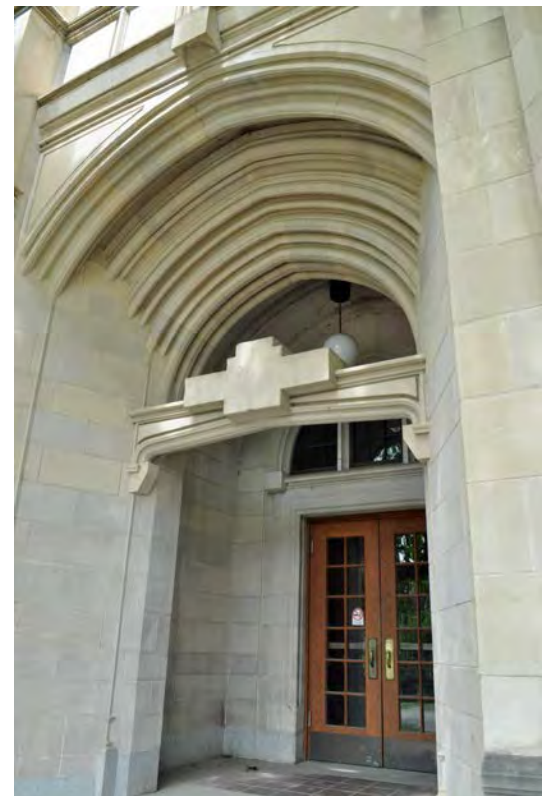
Figure 3. Main entrance to the Physics Building.
