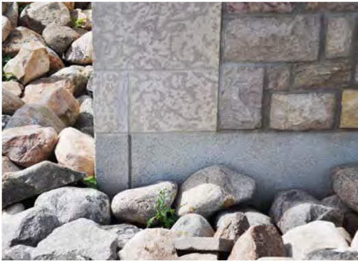
Figure 1. Tyndall stone and greystone above a precast concrete base.
