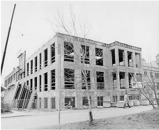
Figure 16. The Administration Building during construction. The concrete walls are visible. Photo A-7037, retrieved from http://scaa.usask.ca/gallery/uofs_events/articles/1956.php
