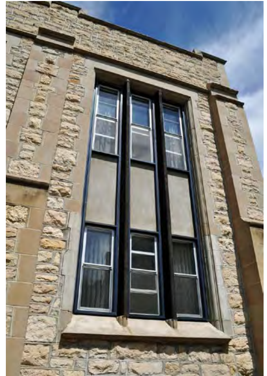
Figure 25. Understated windows on the east side of Saskatchewan Hall.
