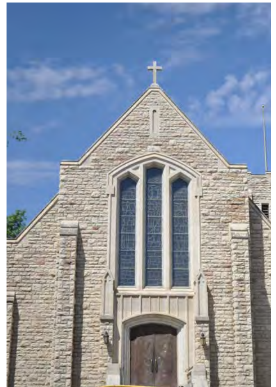
Figure 23. Lancet windows set into a gothic arch formed in stone. Stone piers and references to statuary niches flank the arched entry.
