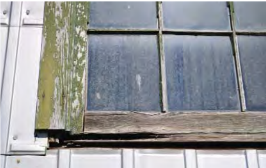
Figure 2. Wooden window frame.
