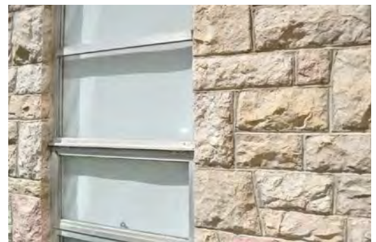
Figure 4. Aluminum framed windows set into a field of greystone.
