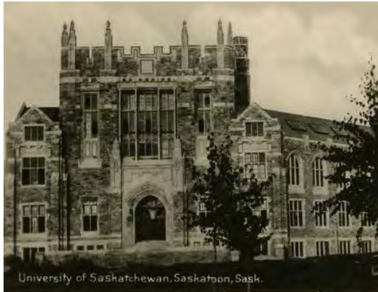
Figure 13. The Thorvaldson Building, ca. 1930. Photo A-10983, retrieved from http://sain.scaa.sk.ca/items/index.php/chemistry-building-5;rad
