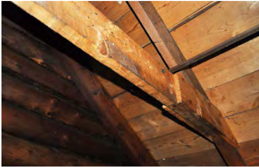
Figure 6. Wooden trussed rafters.
