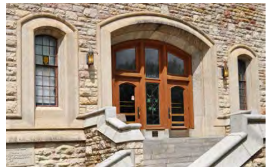
Figure 12. Arched entrance and windows.
