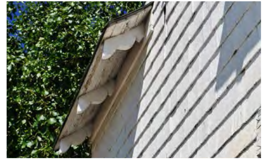
Figure 3. Exposed, profiled wooden rafter ends.
