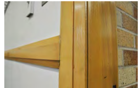
Figure 11. Maple door frame and dado rail.
