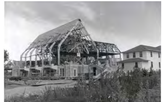
Figure 37. STM under construction, 1953-1956. Photo B.05, retrieved from St. Thomas More College Archives.
