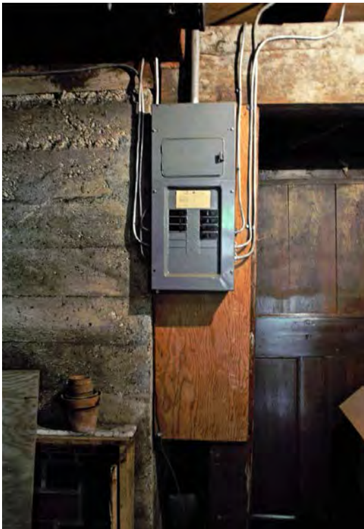
Figure 13. Concrete foundation walls and a wooden post and beam system.
