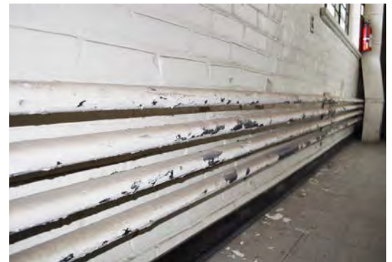
Figure 19. Radiant heating pipes still visible in the Horticulture Building.
