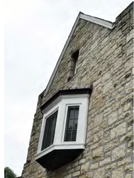
Figure 12. Oriel window with an arched window above it.
