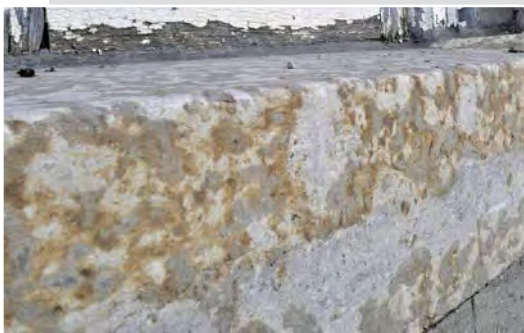
Figure 3. A Tyndall stone threshold.
