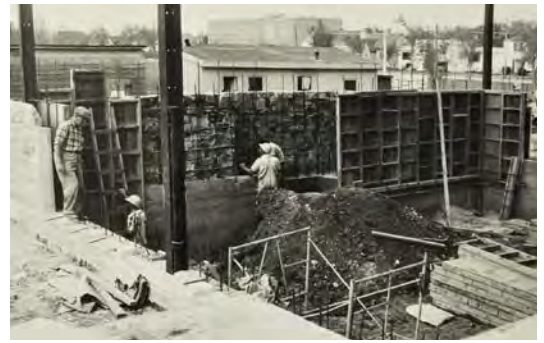
Figure 54. A 1959 construction photo. Photo retrieved from St. Andrew's Archives, File STA.J.21.10.1-43
