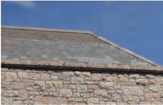
Figure 3. Slate tile roofing.
