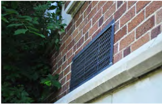
Figure 1. Red brick, artificial limestone and copper grille.
