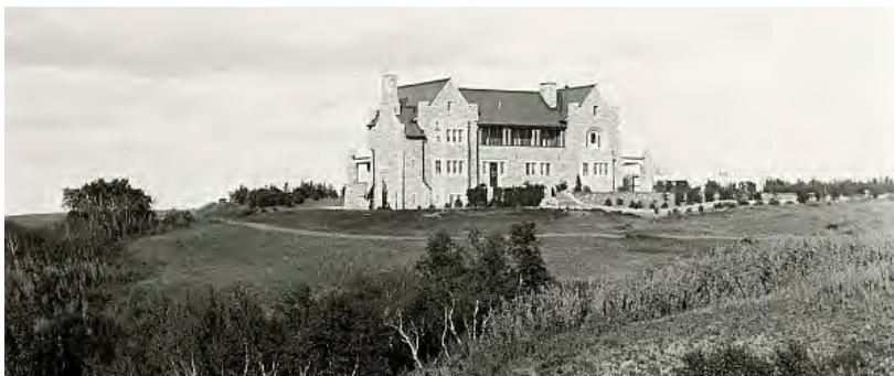
Figure 10. The form of the President's Residence. Photo A-3400, retrieved from http://scaa.sk.ca/gallery/uofs_buildings/
