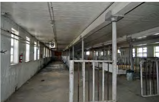
Figure 23. Steel posts support wooden beams.
