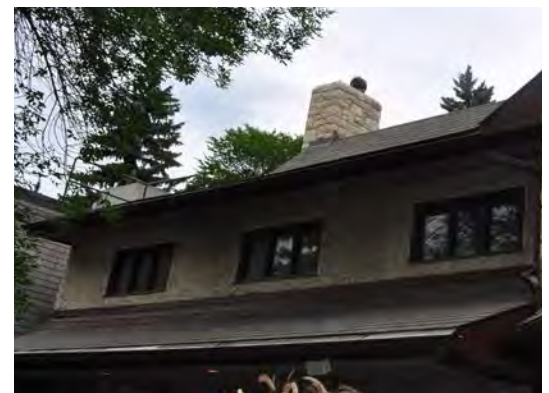
Figure 7. Alteration to former dormer windows.
