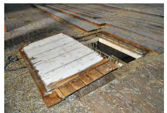
Figure 26. A trap door in the loft opens into an aisle below.
