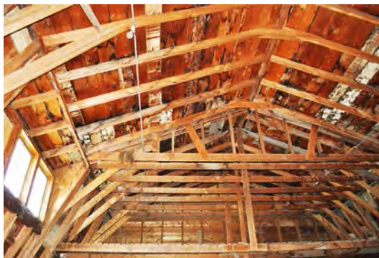
Figure 14. Exposed roof trusses.
