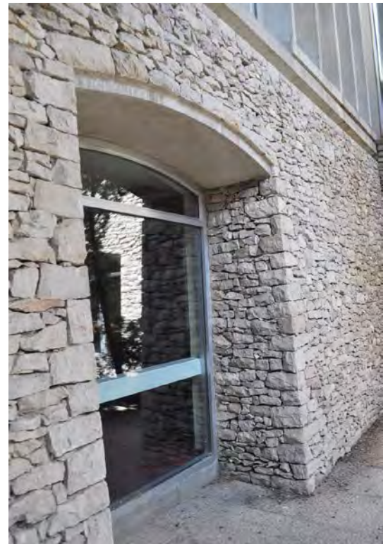
Figure 15. Canted stone wall with arched window openings.
