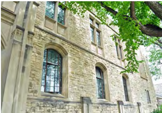
Figure 20. Arched windows, stone piers and spandrels.
