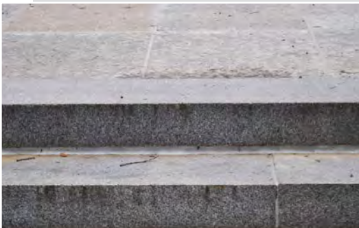
Figure 2. Granite steps and Tyndall stone pavers.
