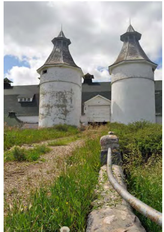
Figure 17. The remaining ramp.
