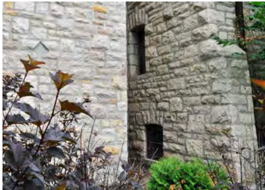
Figure 9. A diamond cut detail on the elevator shaft.
