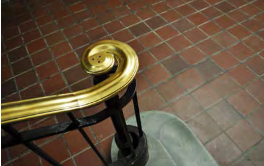
Figure 7. Red terracotta tile, slate stair treads, iron balustrade and bronze banister.
