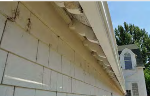
Figure 1. Cedar shingles and exposed wooden rafter ends, both painted.
