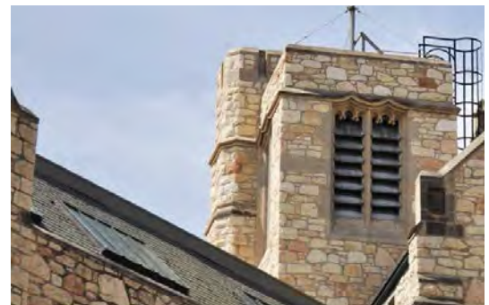
Figure 3. Slate tile roofing, lead covered louvres on exterior venting.
