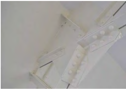
Figure 7. Exposed structural steel.
