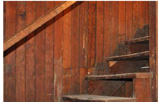
Figure 4. Douglas fir interior walls and stairs.
