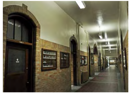
Figure 25. The main corridor of the Physics building relies on electric light.
