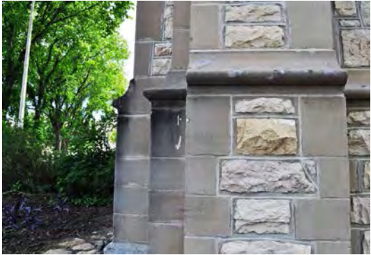
Figure 23. String courses and quoining.
