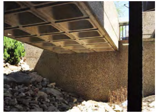
Figure 22. View from basement window.
