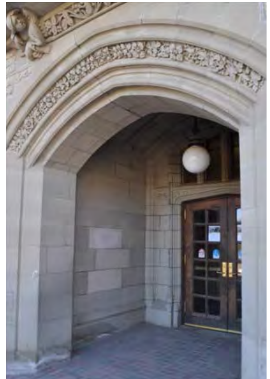
Figure 15. The MacKinnon Building's principle entry recessed within an arch, featuring an arched door.
