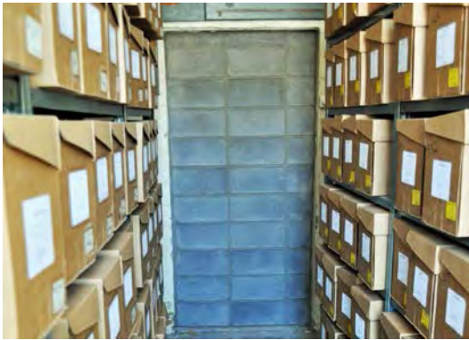
Figure 16. Concrete block fills the openings on the south side.
