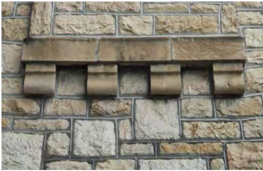
Figure 14. Limestone corbels supporting the underside of a chimney.
