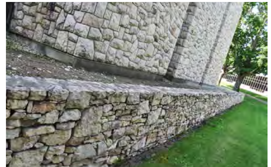
Figure 16. Rusticated greystone base.
