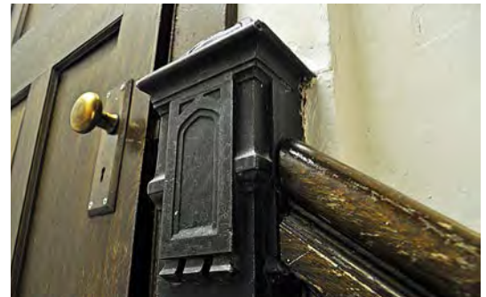
Figure 26. A detail found on all staircases in Saskatchewan Hall.
