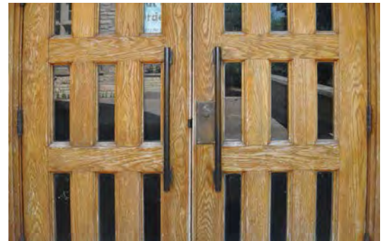
Figure 5. Oak door with glazed panels, brass door pulls, hinges and lock.
