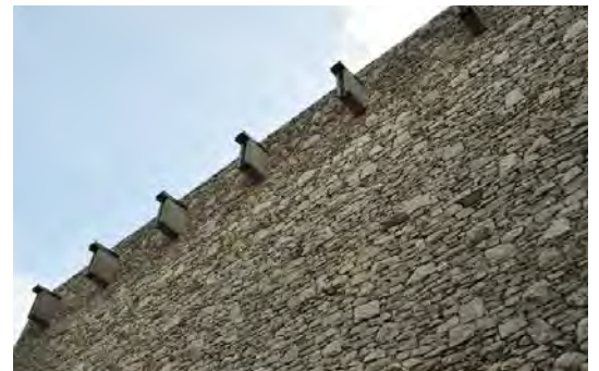
Figure 17. Concrete beam ends on the chapel walls.
