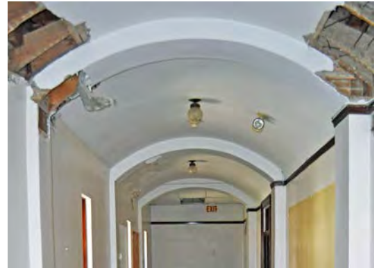
Figure 24. Arched ceiling in the first floor corridor.
