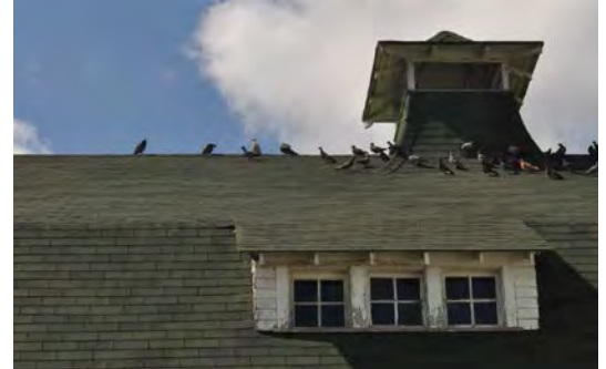
Figure 13. Cupola and dormer window.
