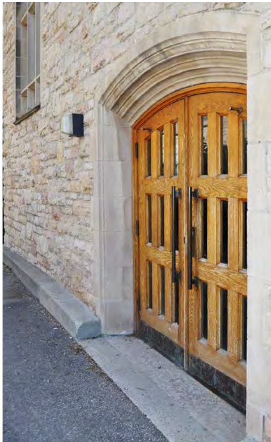
Figure 17. Cut stone arched entrance and doors.
