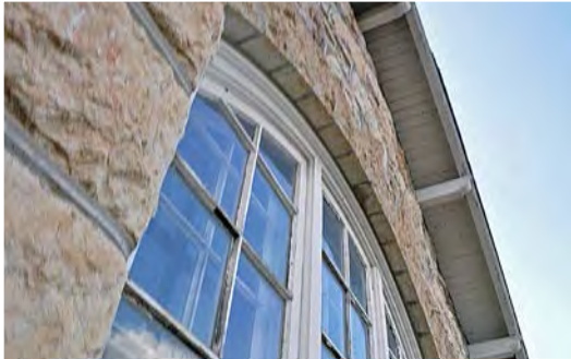
Figure 2. Wood-framed windows in a greystone wall, and exposed rafter ends.
