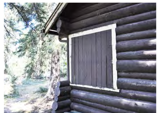
Figure 3. Lindner's studio window with painted shutters nailed shut.
