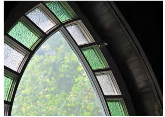
Figure 3. Wood-framed stained glass windows.
