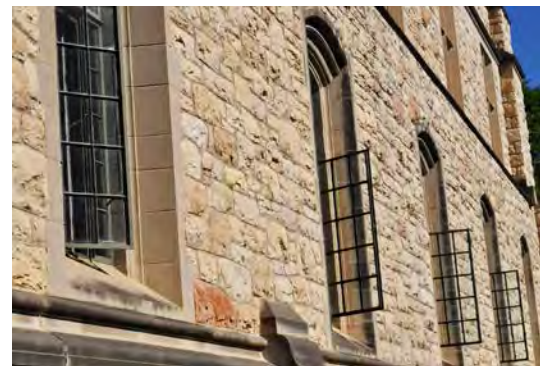
Figure 10. Arched ground floor windows and string courses.
