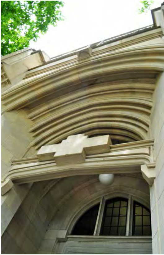
Figure 18. A recessed, vaulted entryway with pointed arches is a Collegiate Gothic character-defining element. Other typical Collegiate Gothic decorative elements, such as grotesques, heraldry and reliefs are absent.
