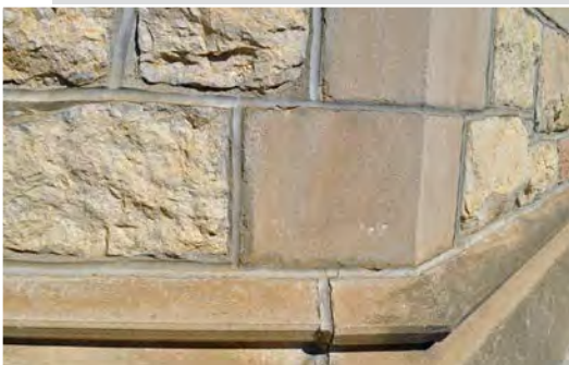
Figure 1. Indiana limestone trim on a 'greystone' wall.
