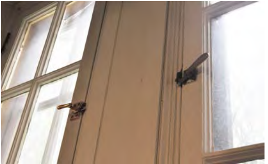
Figure 6. Interior and exterior wood-framed casement windows with brass hardware.
