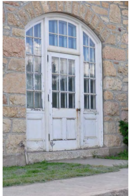
Figure 12. An arched doorway with arched transom and side lites.
