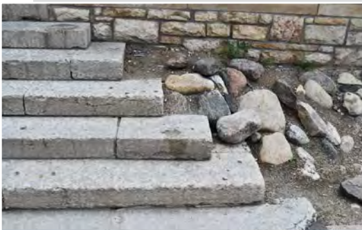
Figure 2. Tyndall stone steps.
