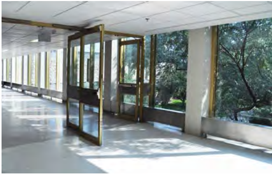
Figure 6. Glazed circulation space.
