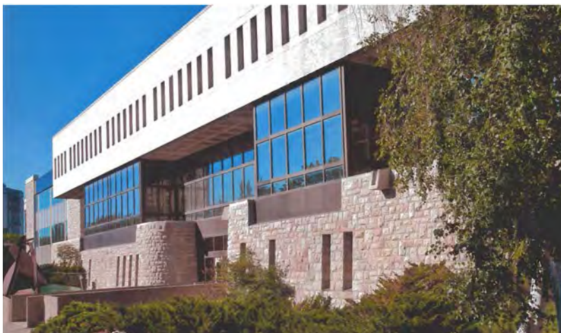
Figure 8. The Dental Clinic. Photo retrieved from Flaman, B. (2013), Architecture of Saskatchewan: A Visual Journey, 1930-2011 .
