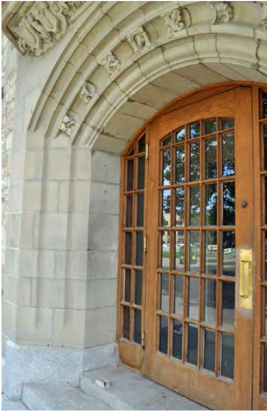
Figure 22. An arched entry.
