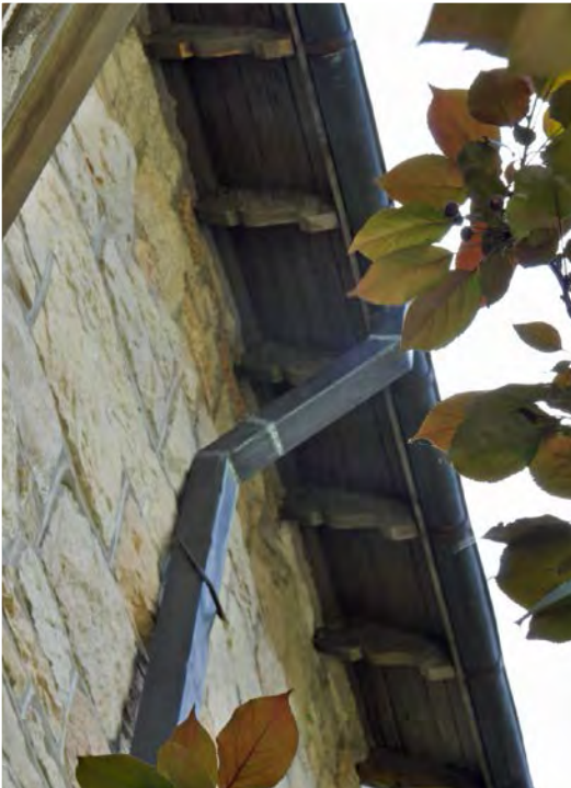
Figure 2. Copper drainage gutter and exposed wooden rafter ends.
