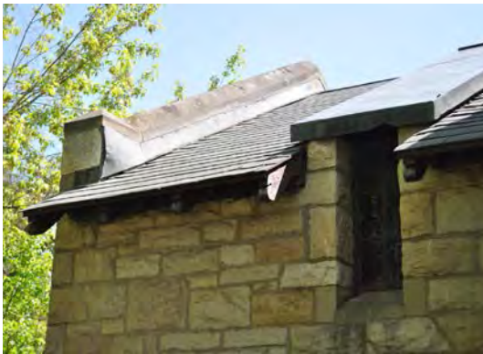
Figure 3. Copper dormer roofing, decorative wooden rafter ends.
