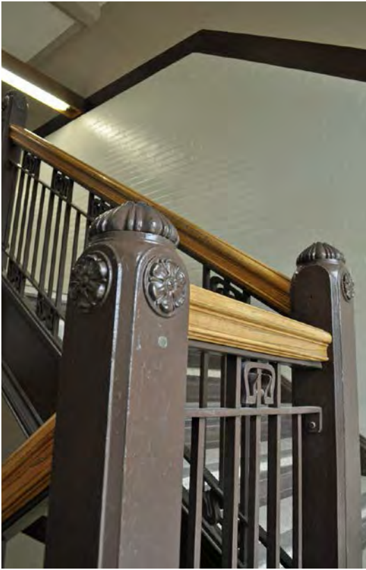
Figure 7. A decorated interior staircase with oak banisters, steel and iron balustrades, terrazo treads and steel risers.
