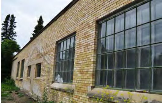
Figure 17. Factory-style windows on the south side of the building.
