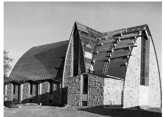
Figure 15. Emmanuel and St. Chad Chapel under construction in 1966. Photo A-346, retrieved from http://scaa.sk.ca/gallery/uofs_buildings/
