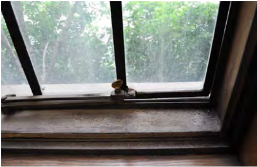
Figure 7. Steel sash window with brass fittings and oak trim.
