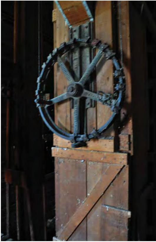
Figure 13. Crank controlling delivery of grain to bins.
