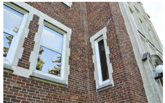
Figure 14. Stone quoins around windows, an archer slot window.
