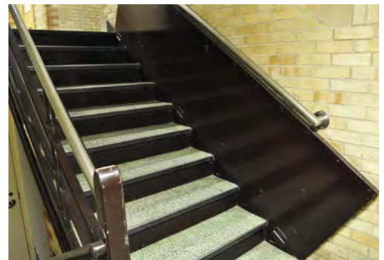
Figure 27. Stair with retractable ramp.
