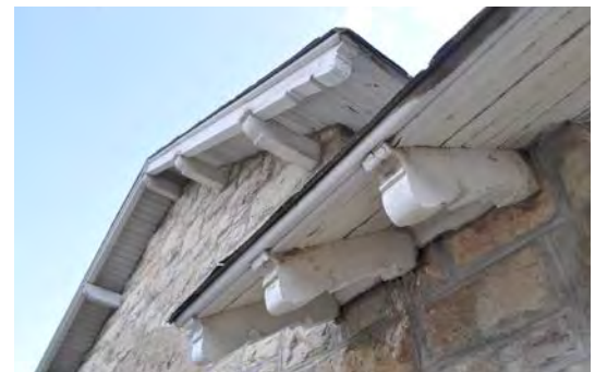
Figure 13. Exposed wooden rafter ends.
