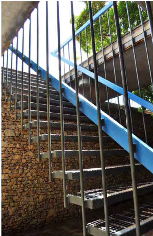
Figure 20. A stair pierces the bridge to the first floor entrance.
