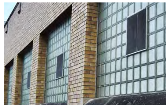
Figure 6. Glass block windows.
