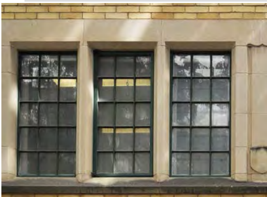
Figure 2. Single glazed steel casement windows.
