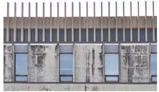
Figure 15. Precast concrete spires.
