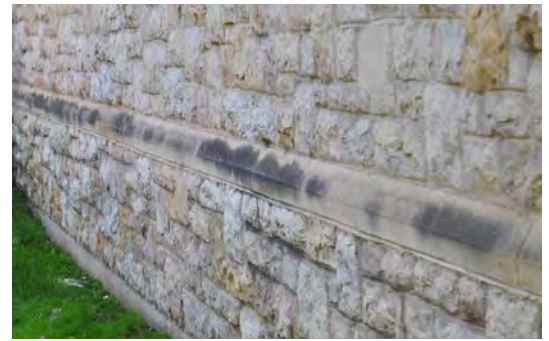
Figure 12. Indiana limestone string course in a greystone wall.
