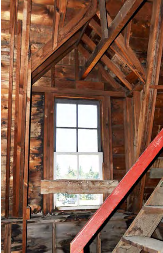
Figure 10. Interior view of peaked dormer.
