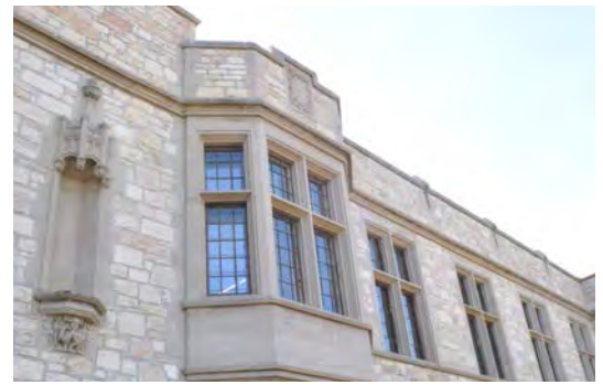
Figure 14. Crenellation along the roofline and an oriel window and statuary niche on the left.
