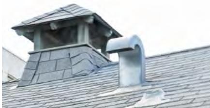
Figure 14. One of two cupolas on the roof of the Horticulture Building.
