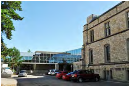
Figure 19. The west side of the building faces onto a parking lot and loading dock.
