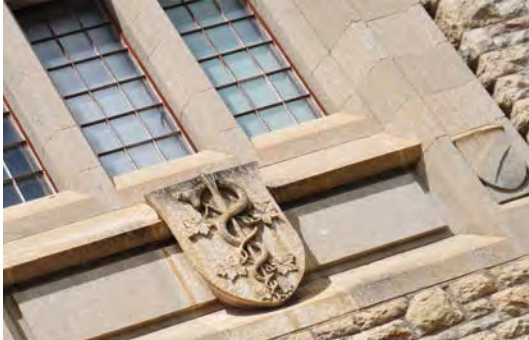
Figure 15. Cut stone medical crest.
