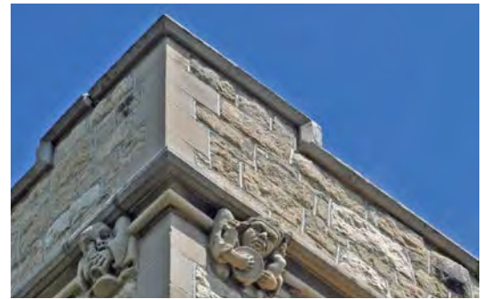
Figure 18. Crenellated parapets define the roofline. Two grotesques are shown, one using a microscope and the other playing a drum.
