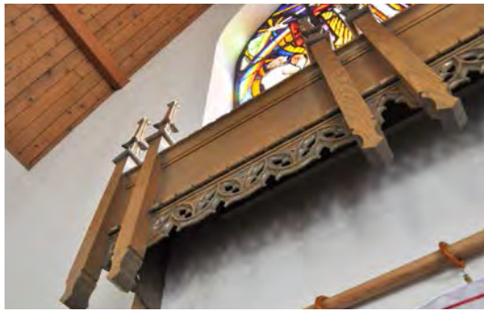
Figure 41. Gothic tracery in the chapel millwork.
