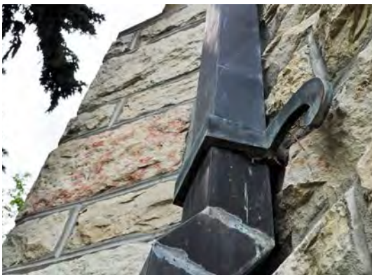
Figure 15. Ornamental bracket on a copper downspout.
