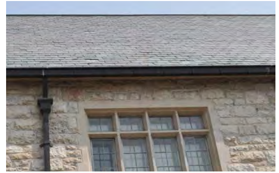
Figure 4. Slate tile roof and copper downspout.
