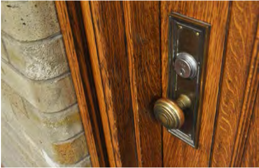
Figure 6. Brick wainscoting, quarter sawn oak door and brass door hardware.
