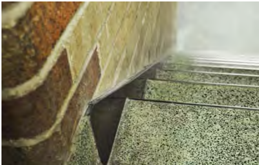
Figure 8. L to R: Interior brick, terrazzo stair treads.
