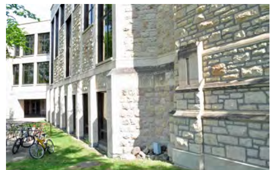
Figure 17. L to R: the facades of the Geology and Physics Buildings.
