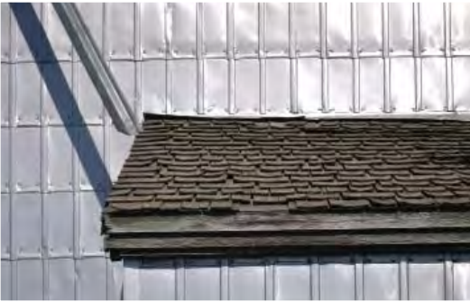
Figure 1. Aluminum cladding, cedar shingles.
