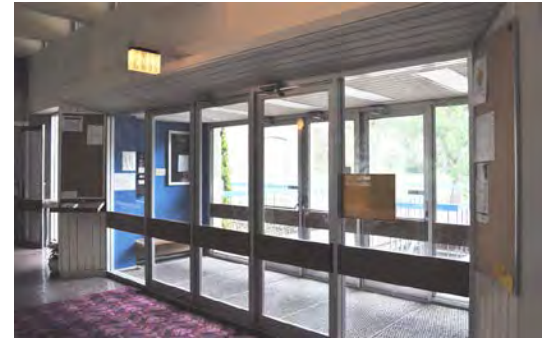
Figure 3. Glazing in the foyer of the Academic College Building.
