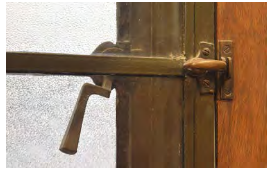
Figure 9. Steel window frames with oak surrounds and brass window hardware.
