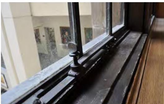
Figure 5. L to R: Steel window frame and fixture with oak sill.
