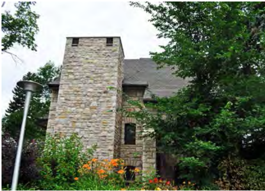
Figure 4. An elevator shaft and the deletion of several windows have greatly changed the eastern facade.
