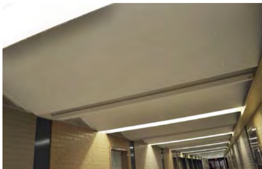
Figure 13. Saw-tooth ceiling in the west classroom wing.
