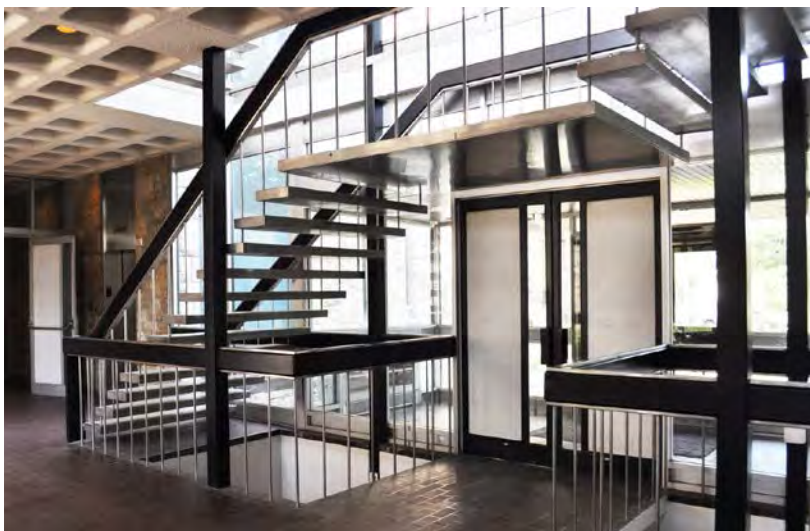
Figure 24. Stair in lobby.
