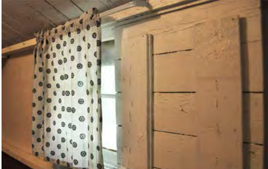
Figure 6. Bedroom window with sliding wooden shutter.
