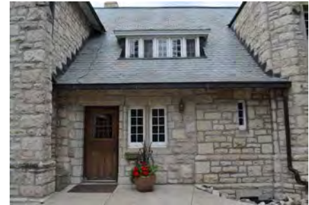
Figure 11. Dormer windows protrude from a roof clad in slate.
