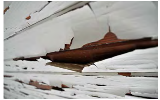
Figure 3. Painted Douglas Fir interior panelling.
