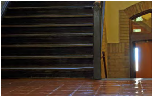
Figure 5. Black slate stair treads and painted clay tile flooring.
