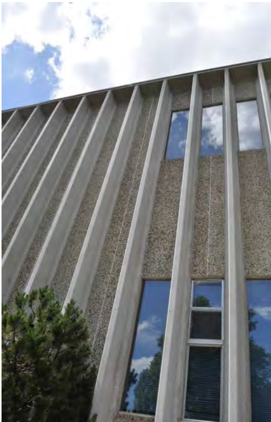
Figure 14. Precast concrete wall panels on the library.
