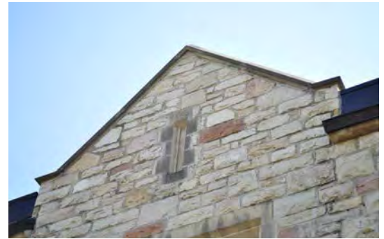
Figure 13. Archer style slot under peaked parapet roof form.
