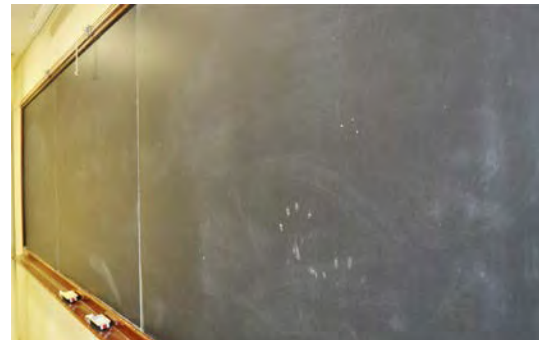
Figure 27. Slate chalkboard in oak frame.
