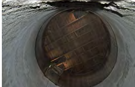
Figure 9. The interior of a silo constructed of concrete and Douglas fir
