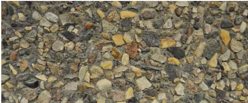
Figure 3. Exposed aggregate concrete.
