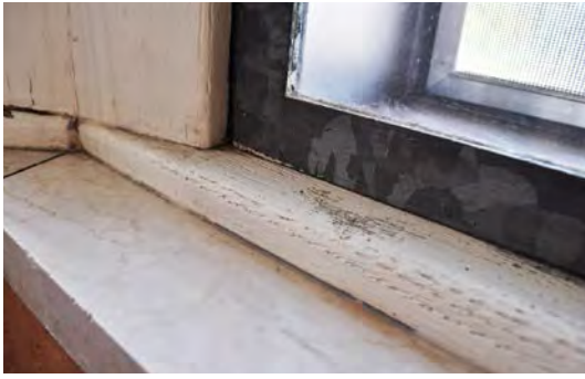
Figure 8. Marble window sill, painted oak window frame and steel sash.
