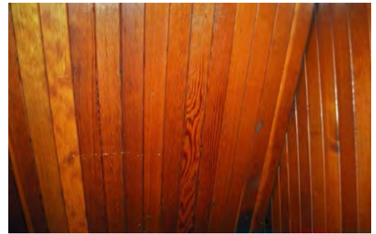
Figure 4. Unpainted Douglas Fir interior panelling.
