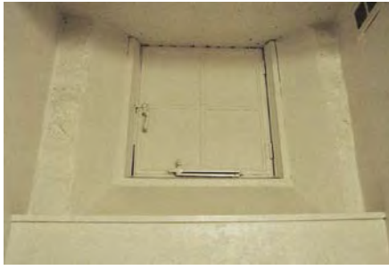
Figure 9. Basement window, painted over.
