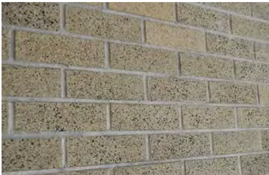
Figure 9. Buff coloured brick.
