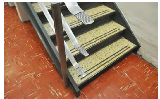
Figure 16. Aluminum balustrade and terrazzo treads.
