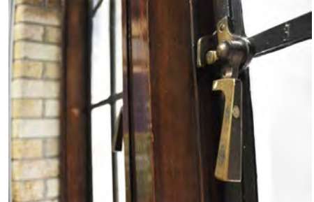
Figure 5. Steel framed window with brass hardware and an oak surround.
