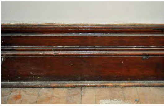
Figure 6. Top to bottom: Plaster wall, oak baseboards, original hardwood flooring.
