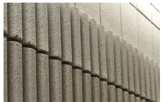
Figure 7. Exposed ribbed concrete block.
