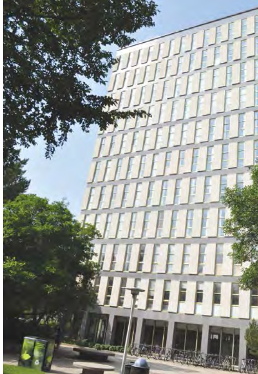
Figure 23. The Arts Tower. The colonnade at the base is clad in grey porcelain enamel. The same material expresses the location of the floor plates above.
