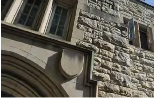
Figure 1. Greystone walls with Indiana limestone trim and decoration.
