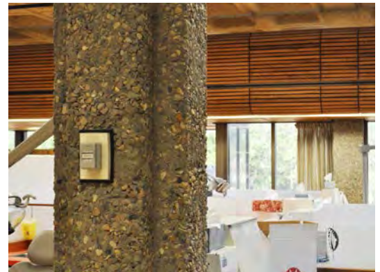
Figure 15. Concrete columns with exposed aggregate finish.
