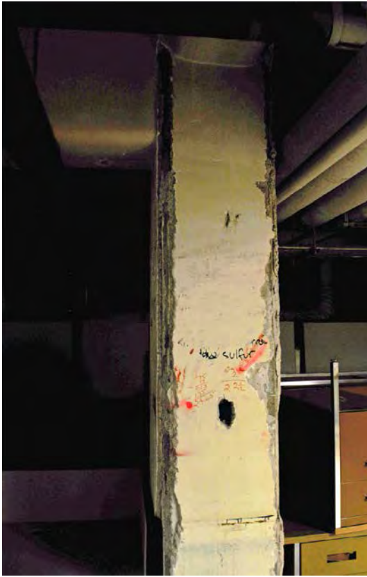
Figure 17. The concrete foundation and footings that withstood the fire of 1925 were reused in the reconstruction of the Engineering Building.
