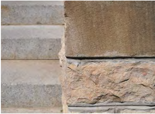
Figure 2. Granite steps, cut limestone trim and greystone wall.
