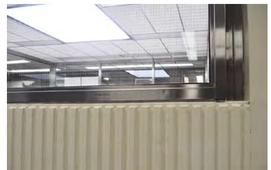
Figure 4. Stainless steel framed clerestory glazing on a painted, ribbed concrete wall.
