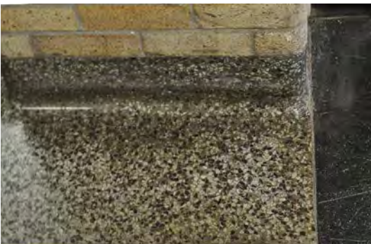
Figure 9. Yellow brick and terrazzo flooring with brass strips.
