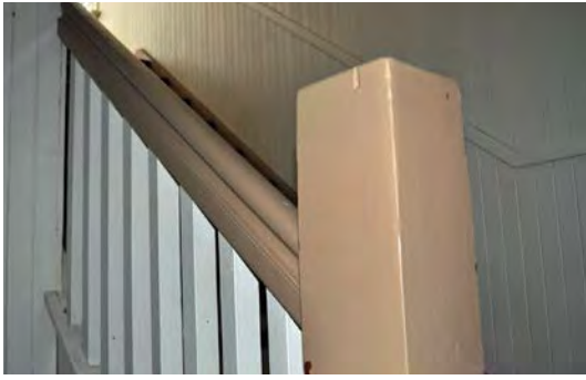
Figure 8. Painted wooden balustrade.
