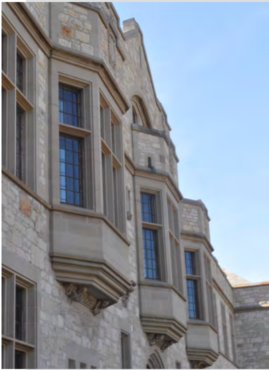
Figure 1. The MacKinnon Building.
