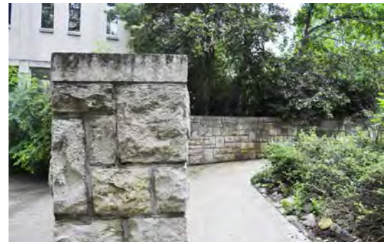
Figure 9. Greystone wall and ramp.
