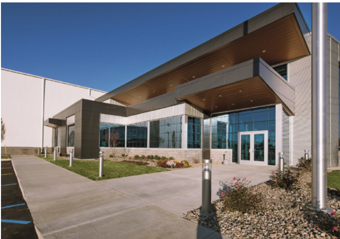
Figure 24. Wood soffit canopy over entrance
