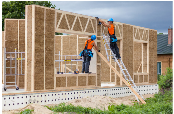
Figure 34. Straw bale construction
