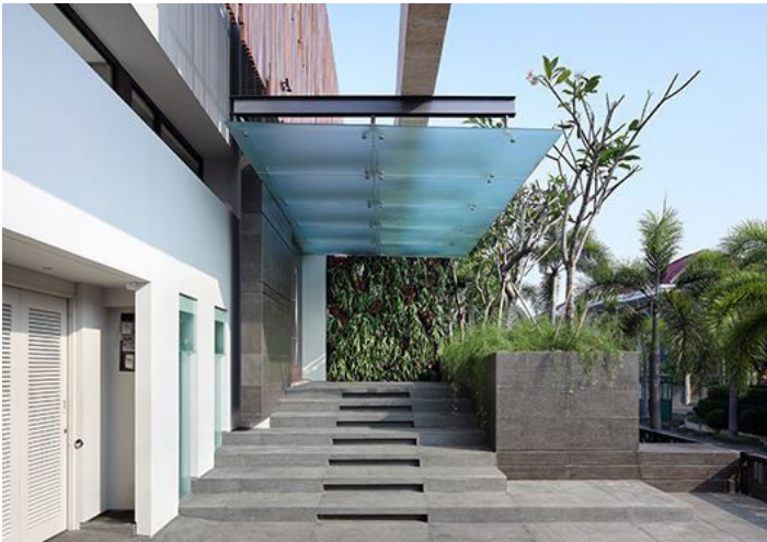
Figure 23. Glazed canopy entrance
