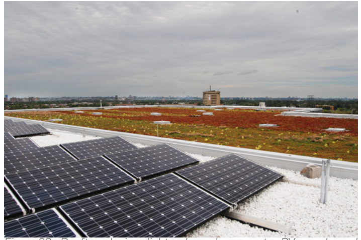
Figure 33. Rooftop design: light coloured aggregate, PV panels and sedum green roof materials
