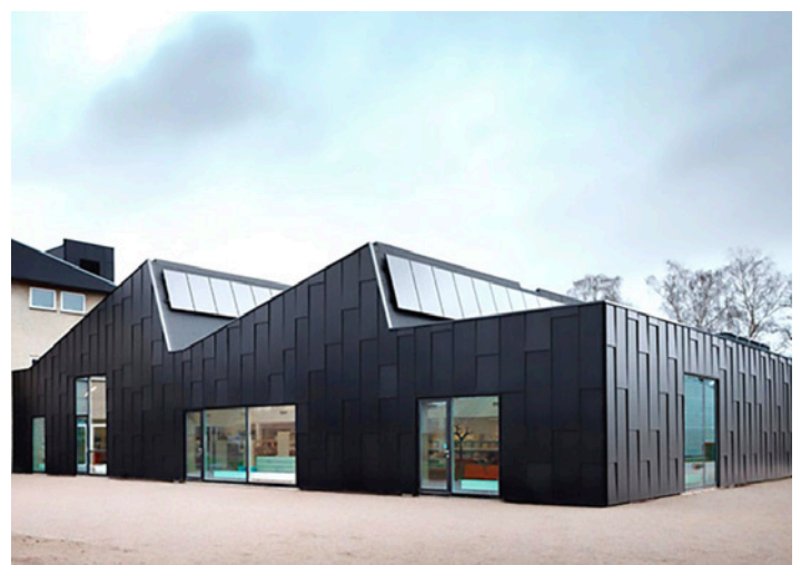
Figure 29. Metal siding, saw tooth roof with PV panels
