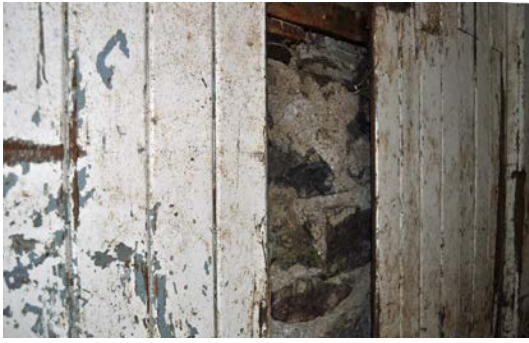
Figure 6. Interior walls clad in wooden planks.
