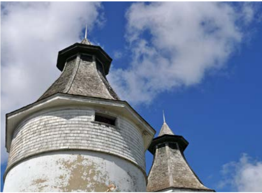
Figure 1. Concrete silos with cedar shingle roofs.
