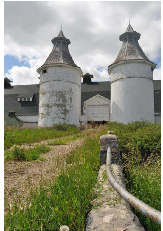
Figure 17. The remaining ramp.
