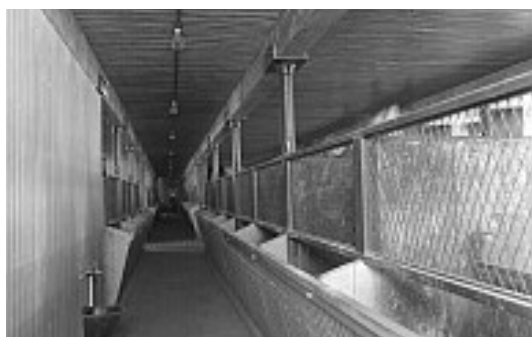
Figure 16. Interior of the horse corridor ca. 1920 with mangers on either side. The photo demonstrates how tightly configured the building was before the stalls were removed. Photo A-72, retrieved from http://scaa.sk.ca/gallery/uofs_buildings/
