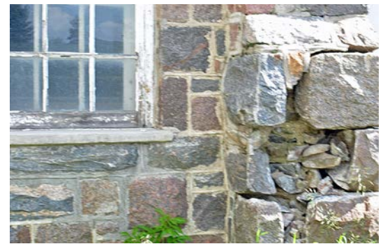
Figure 4. Ground floor walls are constructed of red and grey, rough-faced granite. Windows are framed in wood.
