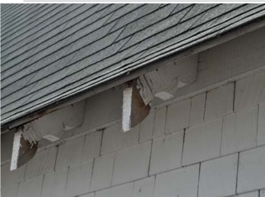
Figure 2. Top to bottom: Asphalt roof shingles have replaced the original cedar shingles, carved exposed wooden truss ends. The cedar shakes on the upper portion of the main barn have been painted white.
