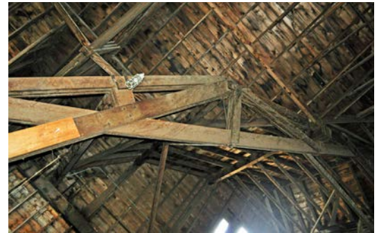
Figure 18. The structure of the barn roof.
