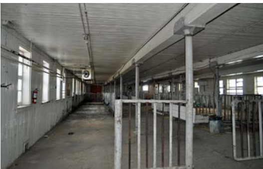
Figure 23. Steel posts support wooden beams.
